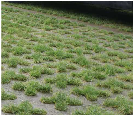
Grasscrete to parking areas
