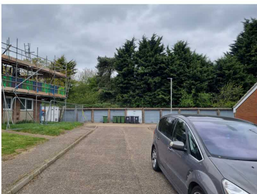
Looking north along access road into site with garages to rear
