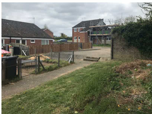
Existing pedestrian link from Green Lane to green space to east, fire damaged flats in background.
